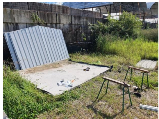
Assembling shed panels
