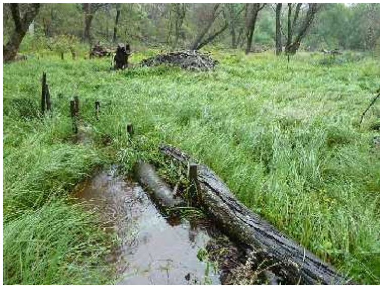
Photo 5. Our structures slow down the flow and disperse it across the silt flat, raising the water table and stimulating growth of the native sedge Carex gaudichaudiana . Note willow stumps, piles of debris and remaining standing willows in background.
